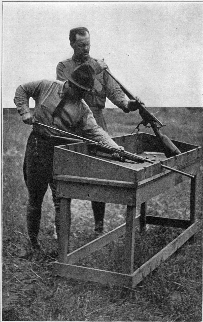
Figure 3. Cleaning rifles, using a cleaning rack
